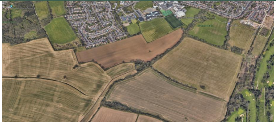
Aerial view looking northwards towards homes on Sutton Close, Oadby.
