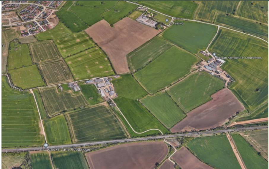
Aerial view northwards of the full extent of the Site.
